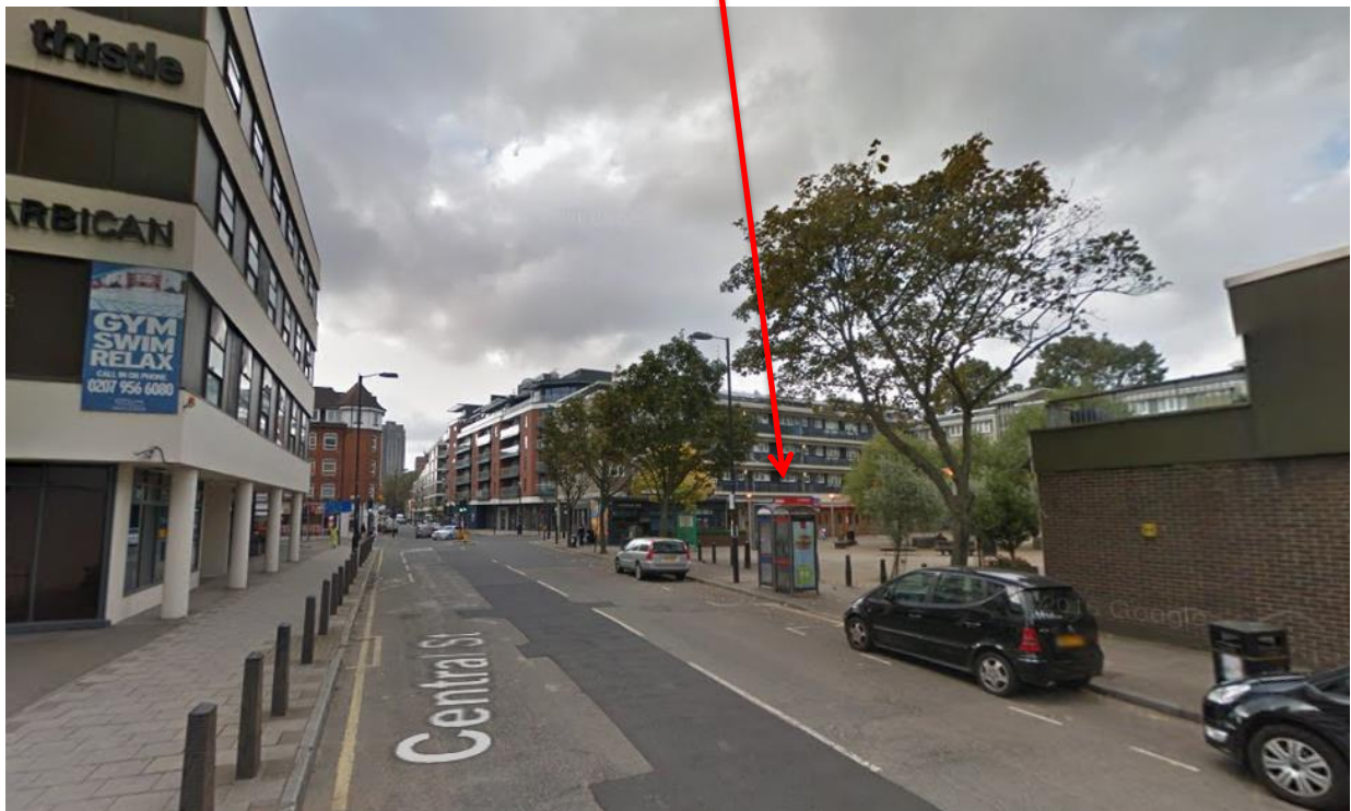
Image 2: View of existing BT phone boxes looking south along Central Street towards Lever Street
